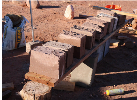
Rammed Earth frame and bricks for the project....
